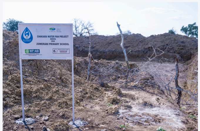
Zowerani primary school waterpan
