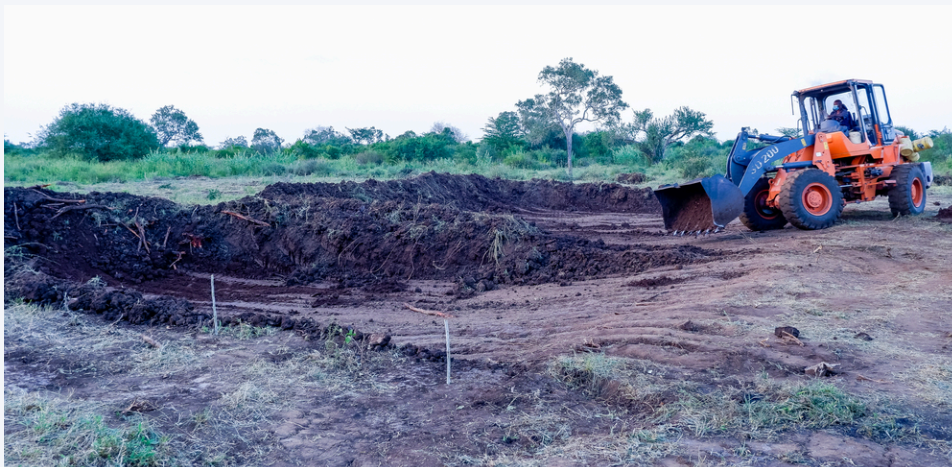
Digging Kibora primary school waterpan
