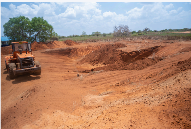
Digging of Chakama secondary waterpan
